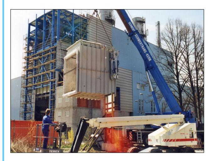
Due to its size the diverter had to be split and delivered to site in several sections, which were then reassembled and placed into position by qualified **RAUMAG – JANICH** personnel. The picture shows the diverter with internal insulation and its hydraulic actuator. The damper is operated by two hydraulic cylinders. Their arrangement ensures that drive shaft bending moments are kept relatively low.
