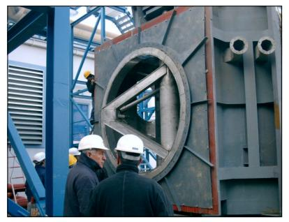
For transportation purposes the diverter was split into several sections. Reassembly on site was carried out under our supervision hand in hand with the customers project management team.
