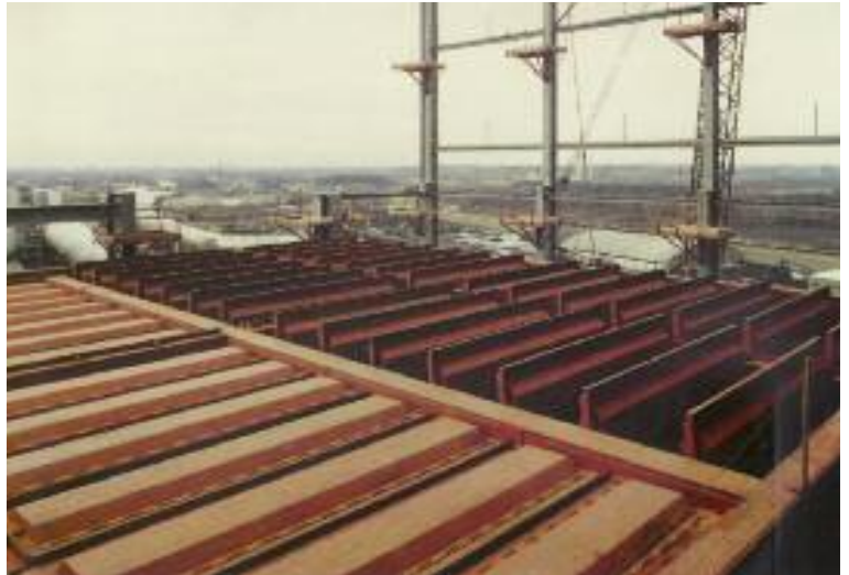
The illustration above shows a shut-off damper for the DeNOx reactor at the STEAG power station Herne 4 . With a nominal size of 16,000 x 17,000mm, it is to date the world's largest shut-off damper.
