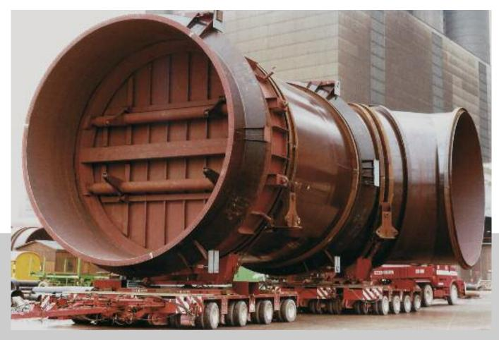
Illustration above: Flap damper DW 7000 mm with duct piece during transportation to the installation site. **FGD at the RWE power station, Niederaussem.**
